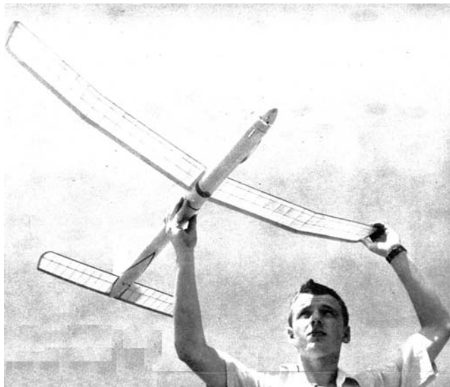
Johnson works with NACA. NACA influence is evident in his attempt at ideal design. Note streamlined stick, squarest wing tips.
